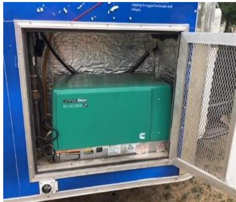
Generator installed in exterior compartment of unit
