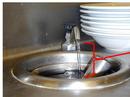
Air gap between water supply line and flood rim of receptacle
