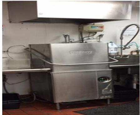
Type II hood over heat/moisture producing dishmachine
