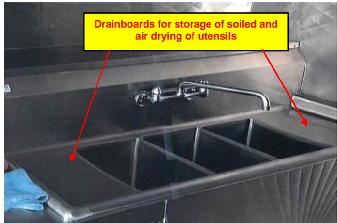
Fixed 3-compartment set up with drainboards
