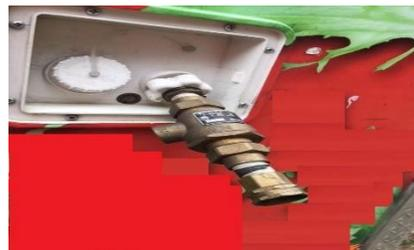
Backflow preventer installed on exterior of unit for connection of public water line
