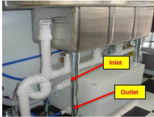
Water tank under 3-compartment sink in unit
